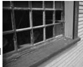
**Photo:** Damaged Window Sill
